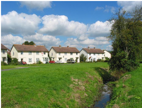
Figure 1: Borough Grove, Petersfield, Hampshire (before refurbishment works)
